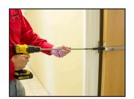
• Connect the 3/8" drill bit to the bullet end drill section.
